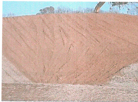
Soils exposed from land grading activities are very vulnerable to erosion
